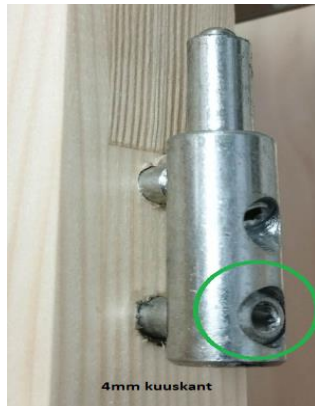
Fig.3 Door sash depth adjustment bolt
