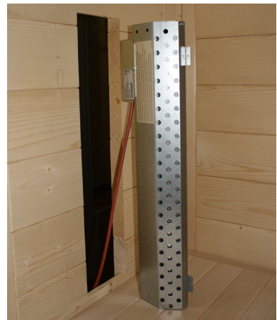
Fig. 2: Terminal box position
