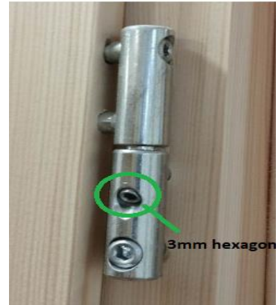
Fig.1 Sash hinge height adjustment bolt
